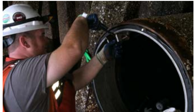
Installing tide valve
