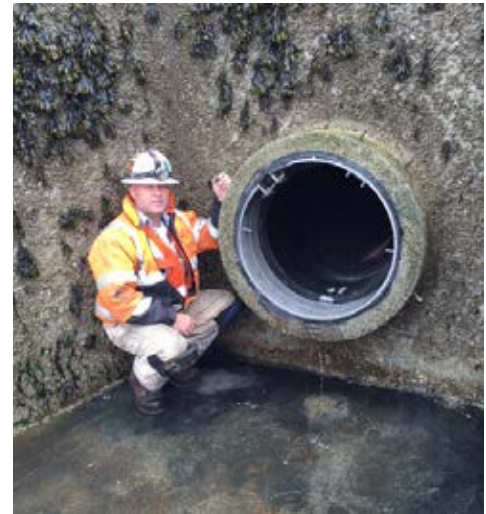
Tide gate inspection at Terminal 10 outfall
